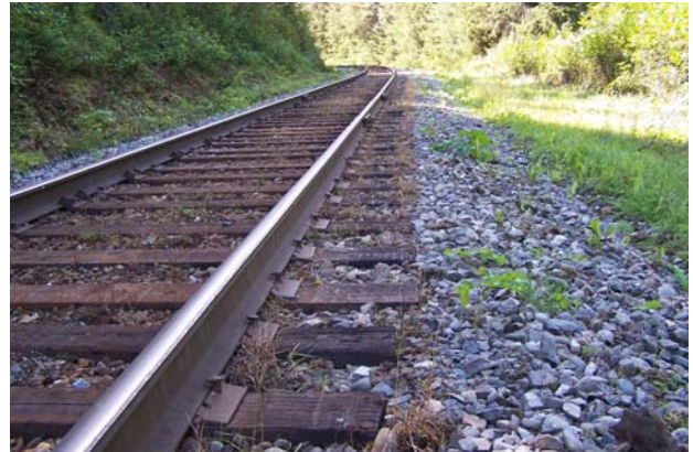
Photo taken several weeks after AquaMaster was applied along the track just north of Seward in July 2010. It illustrates the effectiveness of AquaMaster as a weed-killer, as well as its behavior. The herbicide did not migrate to other areas, but rather only worked on weeds in the tie area where it was applied.
