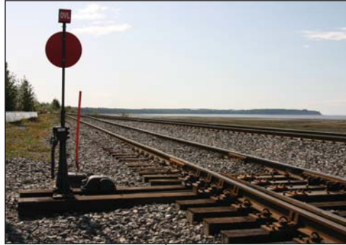
Anchorage Yard southern exit/entrance point.
