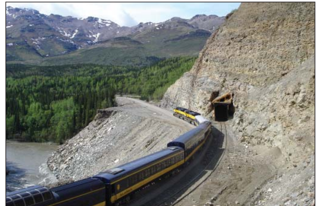
2005: Track is realigned around Garner Tunnel.
