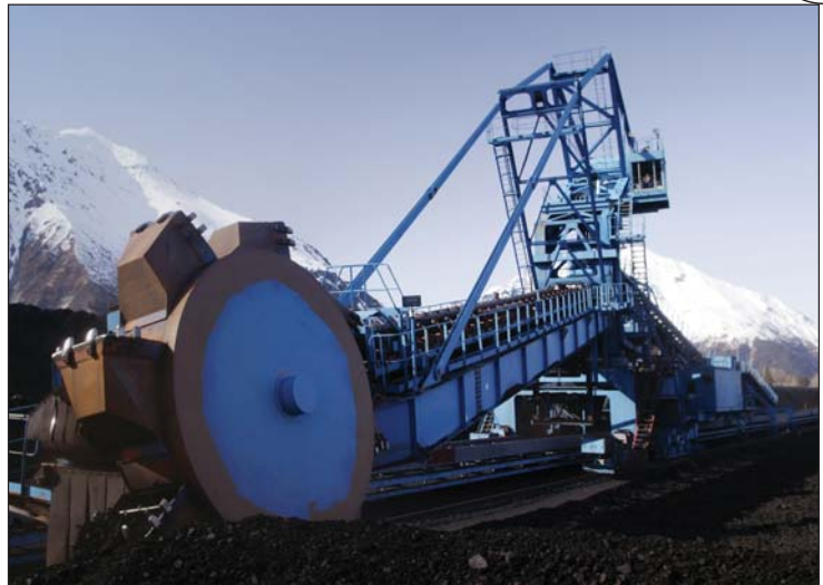
The reclaimer collects coal from the stockpile to put on the conveyor.
