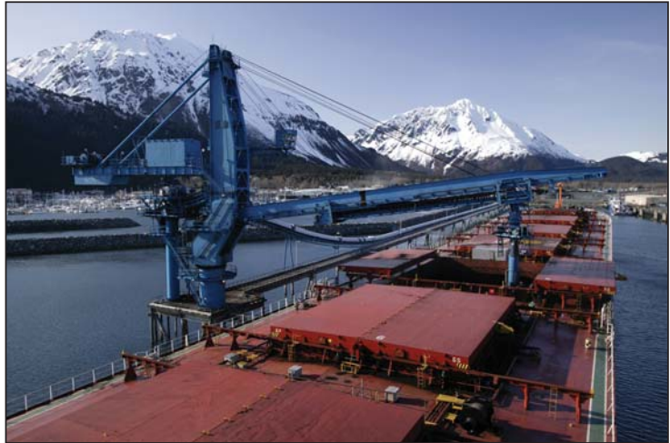
A coal ship loads at the facility's conveyor-fed dock.
