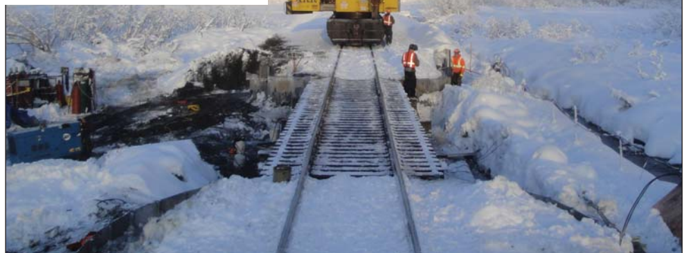
A new bridge was constructed in the Skookum Creek drainage area, and went into service December 2011. A crane was used to drive piling, set the span and backload materials and equipment. Inset: crews weld caps to piles.
