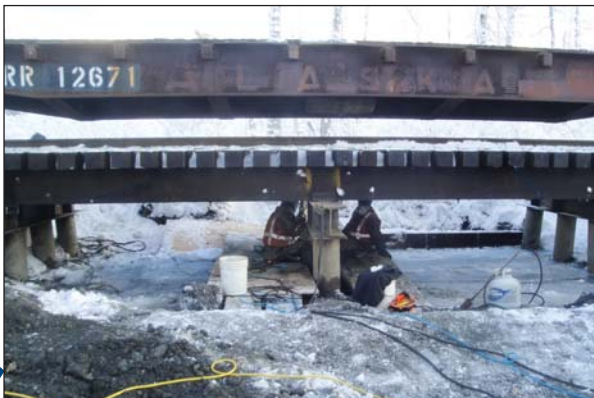
A new bridge was constructed in the Skookum Creek drainage area, and went into service December 2011. A crane was used to drive piling, set the span and backload materials and equipment. Inset: crews weld caps to piles.
