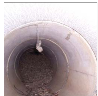
MP 350.8 culvert is blocked.
