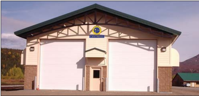
The prototype section maintenance facility built in Cantwell.
