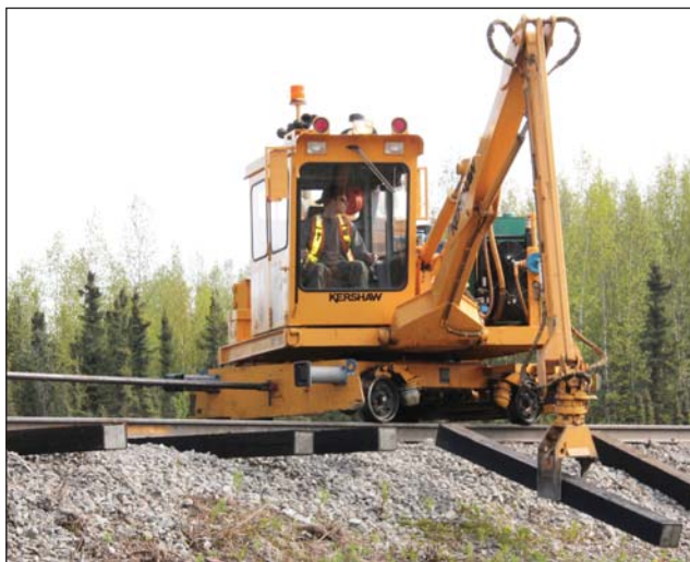
A tie crane operator positions a new tie during tie replacement operations in spring 2011.
