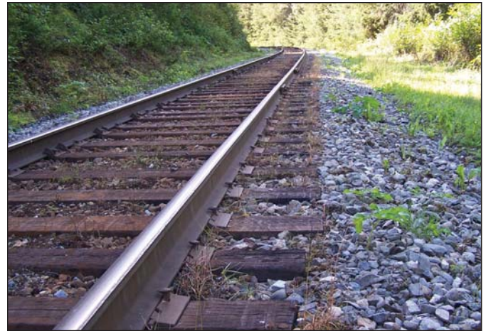
Post herbicide control near Seward. Note clear distinction at control area boundary at the end of the ties.
