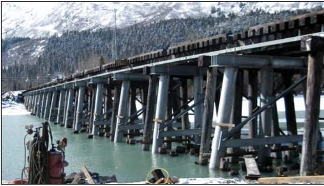
Timber piling and caps were replaced with steel pipe and pile caps on the bridge at MP 29.5 in 2011. In 2012, timber beams and ties will be replaced to complete bridge rehabilitation.
