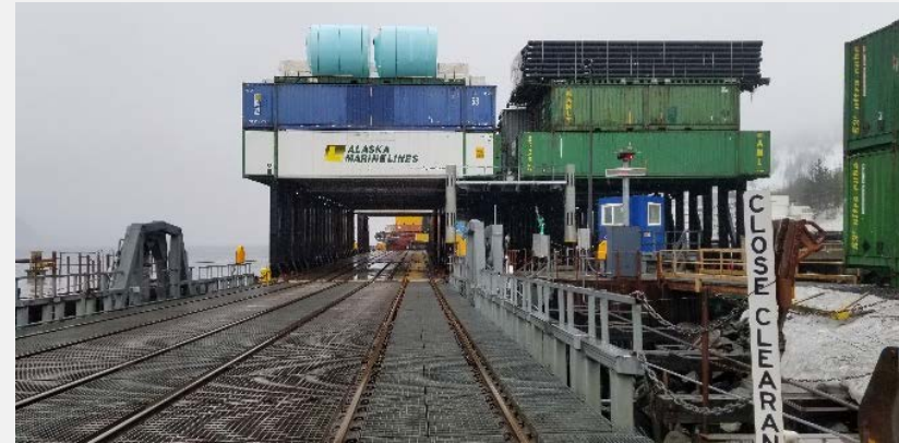
Figure 1: The Barge Slip Connects the Rail Yard to the Rail Barge
