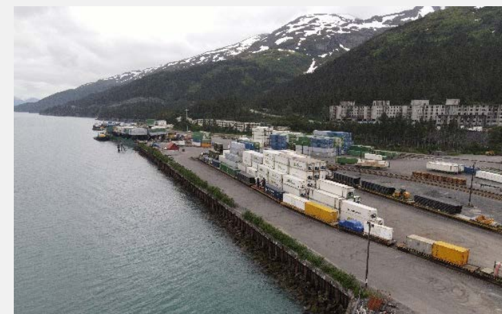
Figure 1: The Combined Intermodal and Manifest Rail Yard and Container Storage
