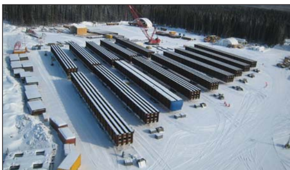
Left: Aerial photos taken by ARRC Board Director John Binkley in late March 2013 show bridge construction activity. Top: progress made on the bridge pier foundations. Bottom: Girders are bolted together into spans in the construction yard. Spans will eventually be set upon the piers.
