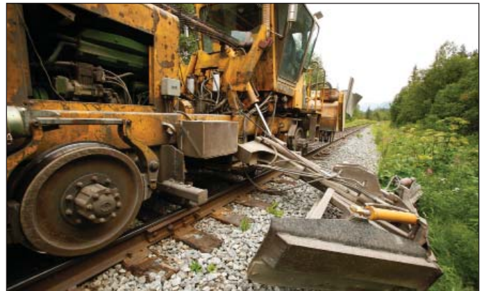
A ballast regulator is equipped to scrape weeds along the side of the track bed, which tempers weed growth temporarily.
