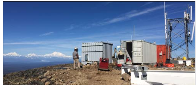
A new communication site is erected on Bald Mountain.
