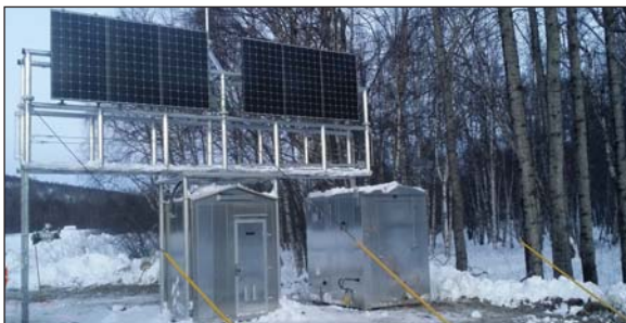
Wayside equipment at Curry is housed in new shelters and powered by solar energy generation and solid oxide fuel cell technology.
