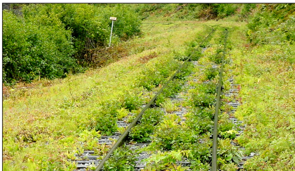
Overgrown weeds on the track are nearly impossible to eliminate with non-chemical methods.
