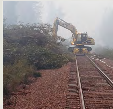
An excavator clears felled trees along a wildfire-scorched, smoke-clogged area.
