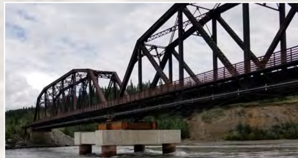
The project to replace the center pier on the bridge over the Nenana River at MP 370.7 was completed in 2019. Bridge infrastructure was damaged during the floods of 2012.
