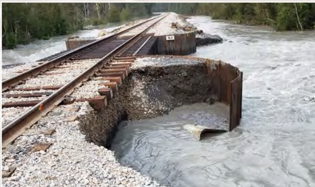
High water on Snow River scours bridge infrastructure along the track between Moose Pass and Seward.
