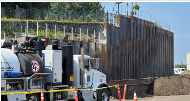
A new retaining wall along Christensen Drive is completed during summer 2019, creating more space to build a commercial roadway west of the Anchorage Historic Depot.
