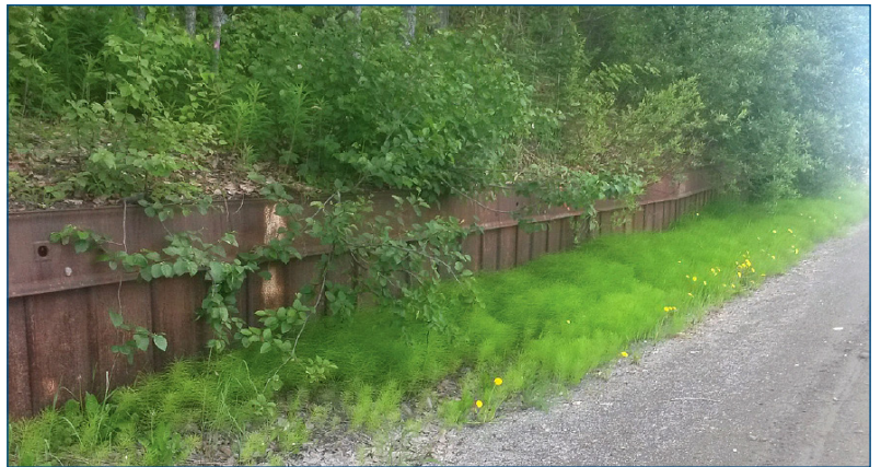
The project will replace the existing retaining wall.
