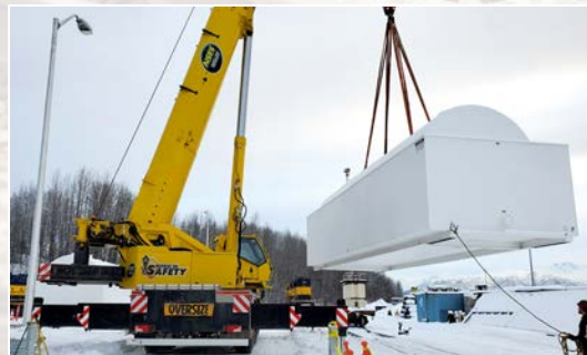
A modern above-ground fuel tank is placed, as part of the Anchorage Yard's new locomotive fuel delivery and control system completed in May.
