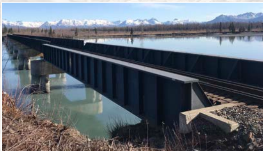
Rehabilitation of Bridge 146.4 over the Knik River was completed in 2020. The railroad received several federal grants in 2020 that will support bridge replacements and rehabilitation work in 2021.
