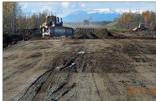
Segment 5 grade work in September 2015.
