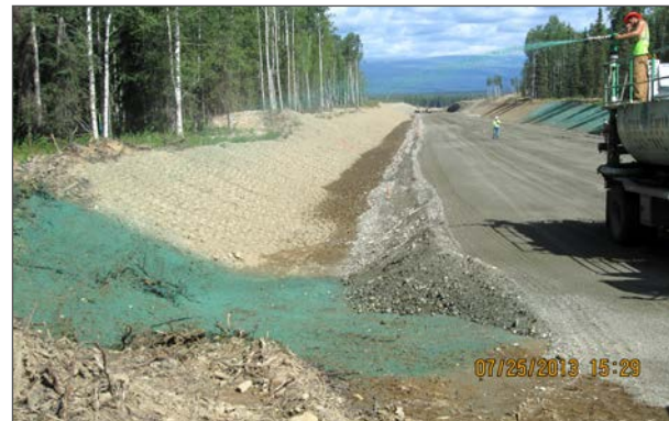
Seeding new embankment along Segment 6 in July 2013.
