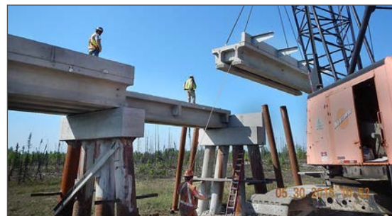
2015 Segment 4 grade work on trail relocation.
