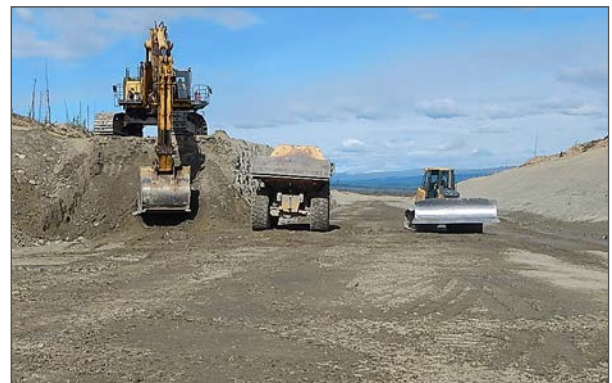
August 2015: Machinery at work on Segment 5.
