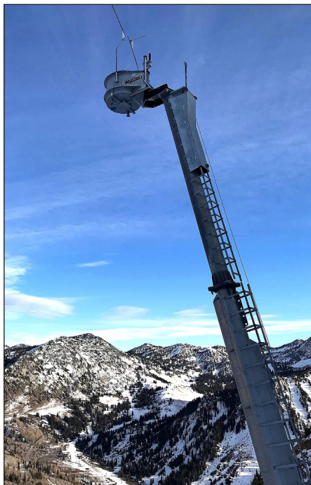
Example of Hanging Charge Control Tower
