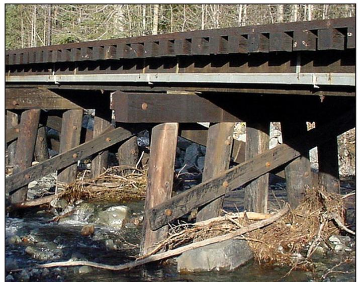
**Project work will include full replacement of the existing bridge. Left: a project drawing shows greater detail on replacing the bents and piles. Right: the photo shows existing bent-and-pile structure.**
