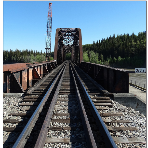
Looking at Bridge 370.7 over the Nenana River from the south-end abutment.
