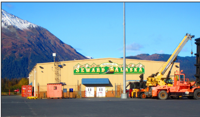
The terminal building sits on the north (land) side of the West Dock. This view is from the water end of the dock.
