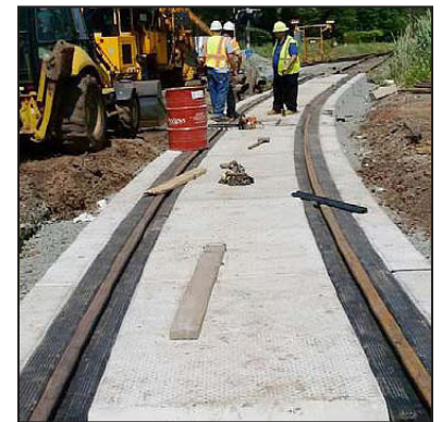
Rail flangeways filled with rubber.
