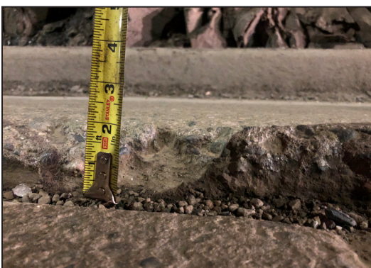
Left: An example of a dip in a concrete panel that requires repair. Above: a graphical explanation of how dips and voids in concrete panels are filled and patched to ensure a surface profile that is even and at the correct height.
