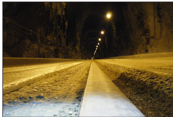
Rail flangeways filled with asphalt.
