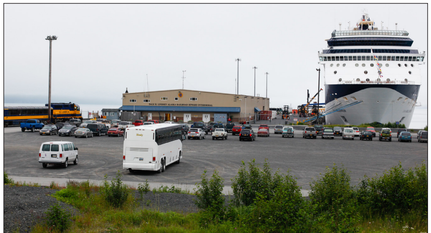
The existing dock and terminal building serve as an intermodal hub, with bus, train and marine connectivity. The dock structure is nearing the end of its useful life.
