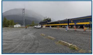
The existing passenger platform will be relocated south and expanded. Limited gravel parking areas will be expanded, paved and striped.
