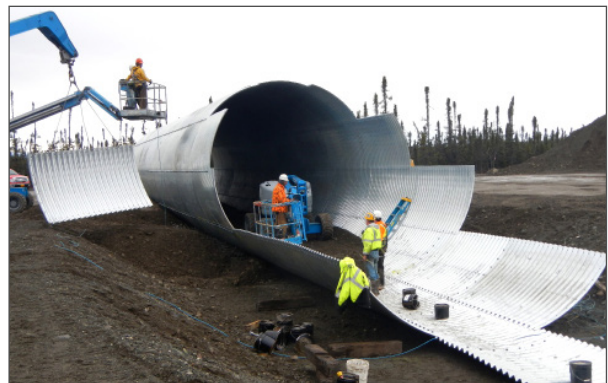
Building a Segment 1 winter trail culvert crossing fall 2013.
