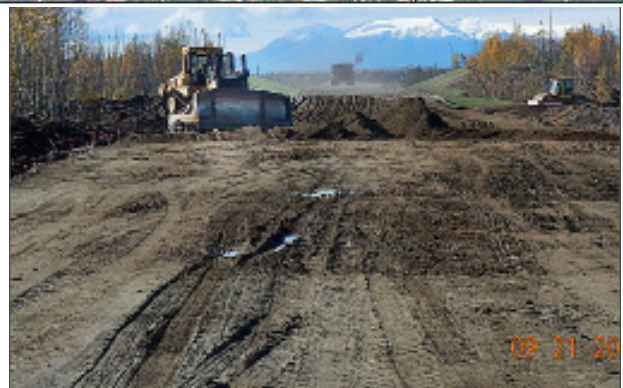
Segment 5 grade work in September 2015.
