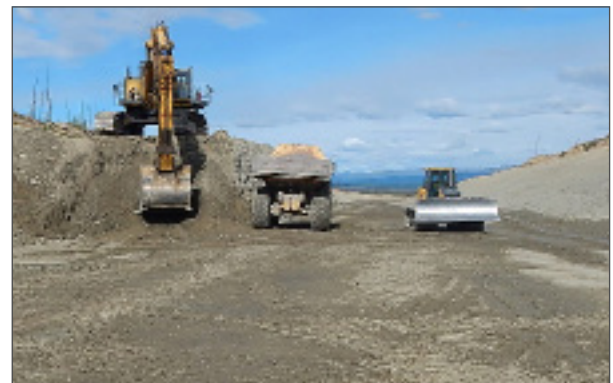
August 2015: Machinery at work on Segment 5.
