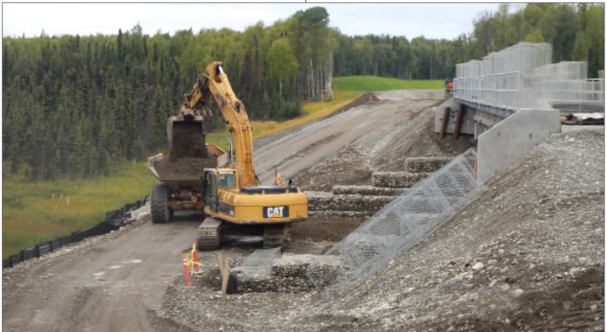
Segment 4: 2015 summer work on a 140-foot 5-span concrete girder bridge over a tributary to the Little Susitna River.
