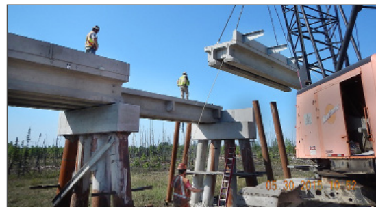
2015 Segment 4 grade work on trail relocation.
