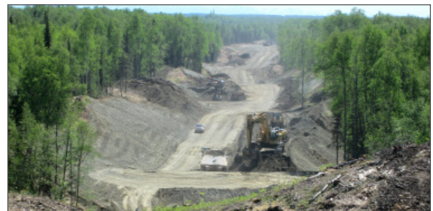
2013 Segment 3 grade work north of W. Susitna Parkway.
