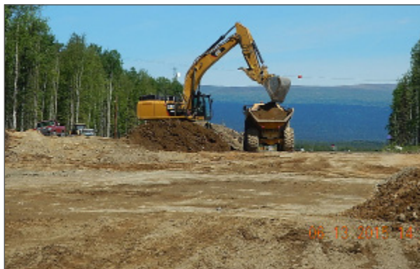
Segment 5 grade work June 2015.
