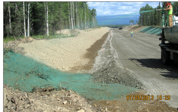
Seeding new embankment along Segment 6 in July 2013.
