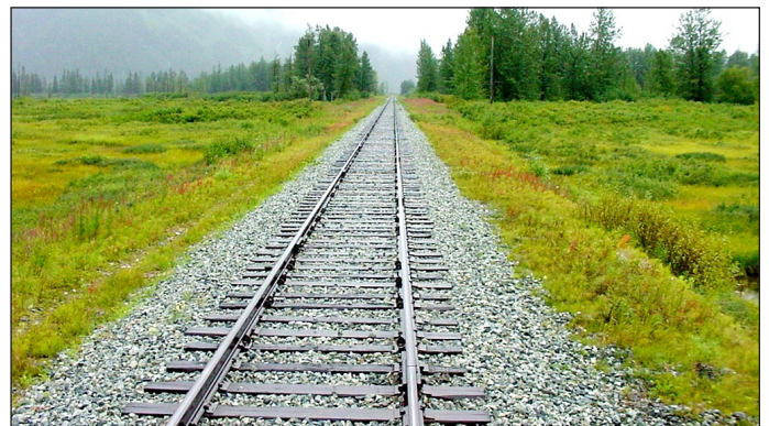
Optimally, the Alaska Railroad track would be free of weeds, providing an uncompromised platform for train movement.
