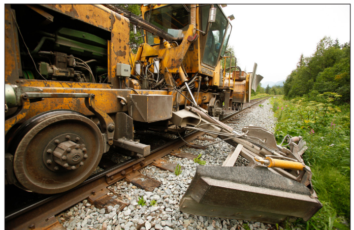
A ballast regulator is equipped to scrape weeds along the side of the track bed, which tempers weed growth temporarily.
