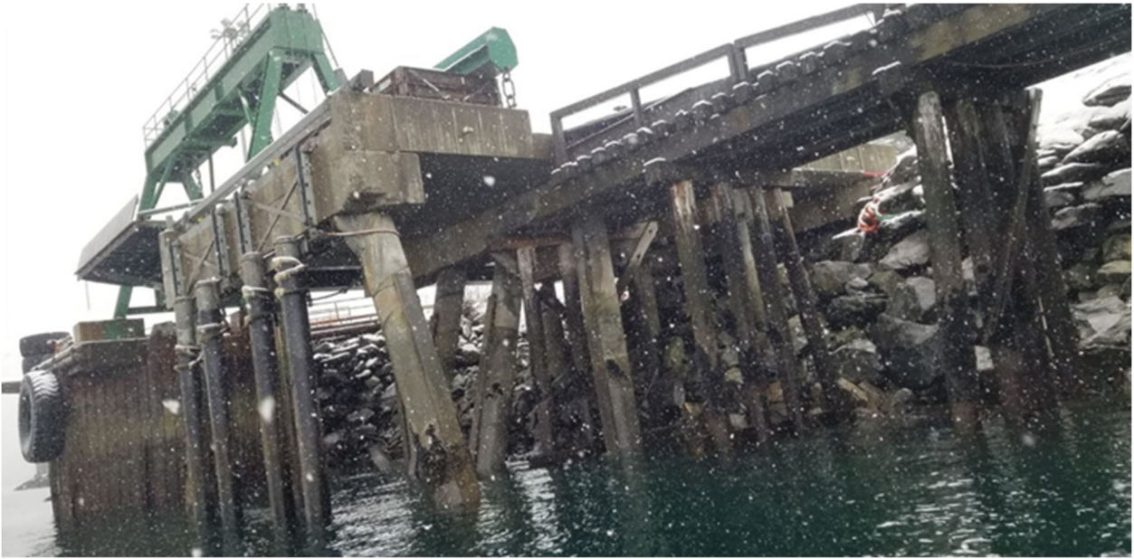
Figure 22. Barge dolphin (left) with fendering and transverse loading ramp within the barge slip.
