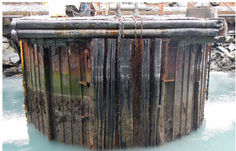
Figure 5 - Sheet piling highly corroded and damaged
