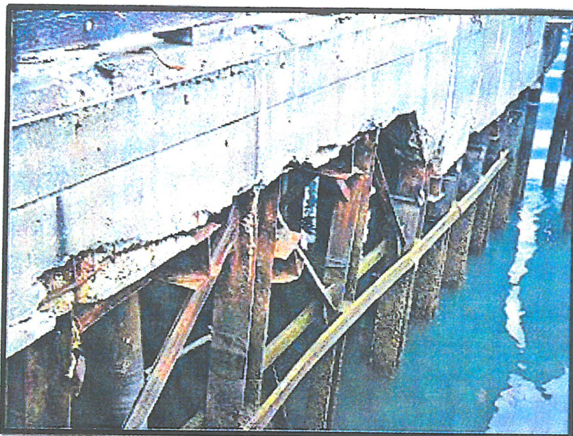
Photo 3: Marginal Wharf: corroded piles and damaged cap
