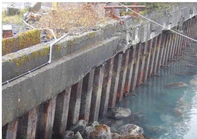
Figure 3 - Marginal Wharf Bulkhead Wall
