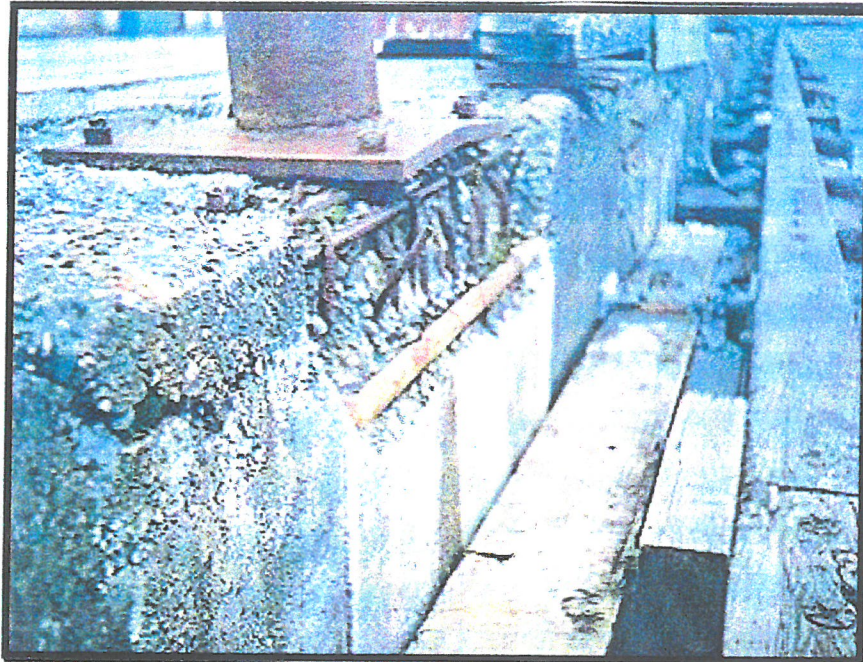
Photo 5: Marginal Wharf: exposed reinforcement in pile cap
