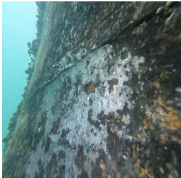
Image 7 – Knife Edge Corrosion Pile Weld
