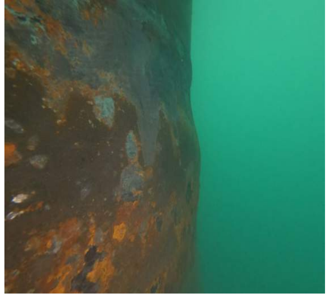
Image 2: Bulbous Deformation
