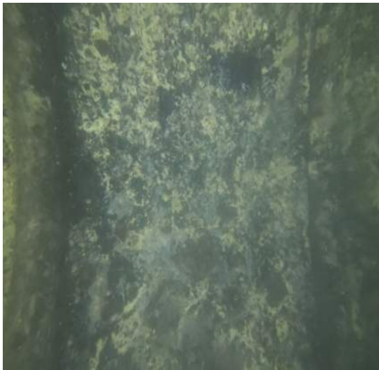
Image 13 – Typical Medium Corrosion
