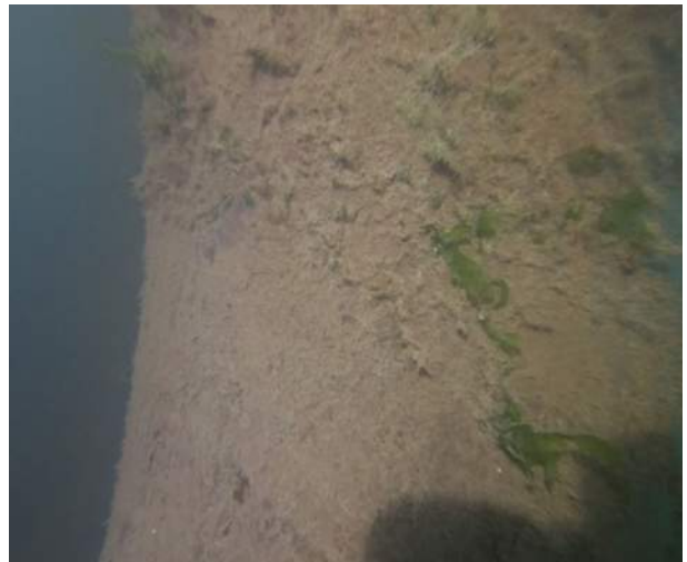
Image 27 – Typical Pile Light Growth
