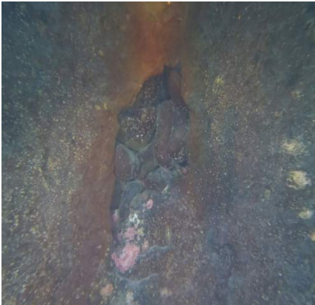
Image 6 - 10"x5" Hole, West Side Cell
