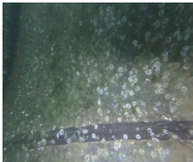
Image 25 – Trestle Steel Pile, Typical Condition
