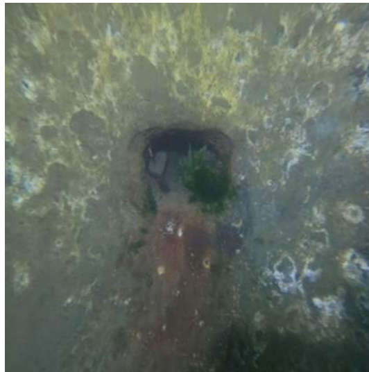
Image 14 – 3" Hole found (Corroded Tieback?)
