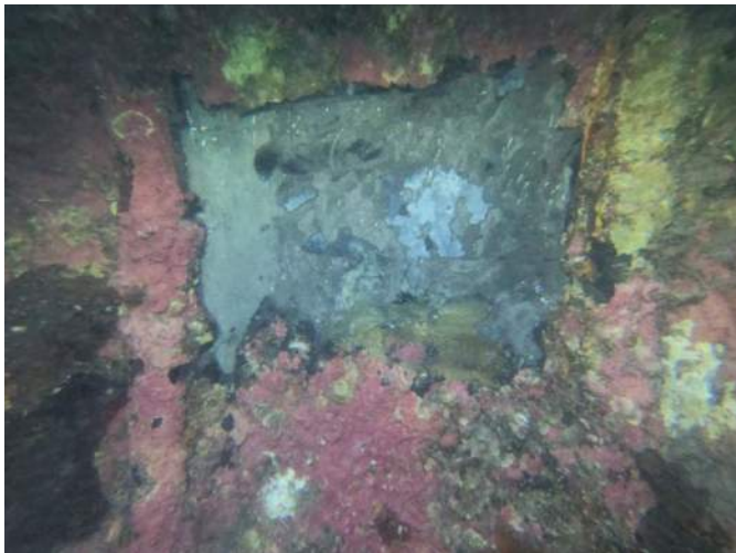
Image 16- Heavy corrosion, pitting and material loss
