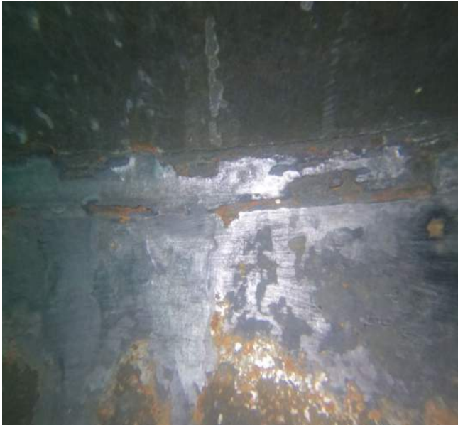
Image 1: Heavy Corrosion
