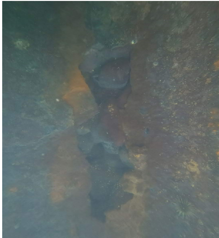
Image 3 - 4" x 18" Hole North Side of Cell
