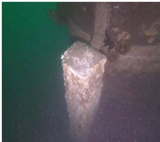
Image 23 – Close up of anode end
