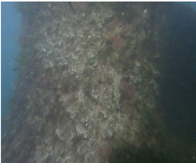
Image 28 – Typical Pile Growth near surface
