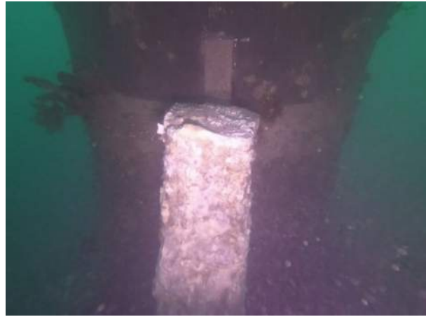
Image 22 – 2020 installed anode typical
