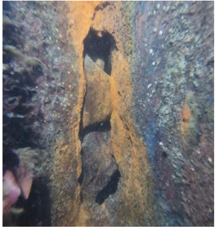
Image 19 – 4" x 11" Hole, South side cell
