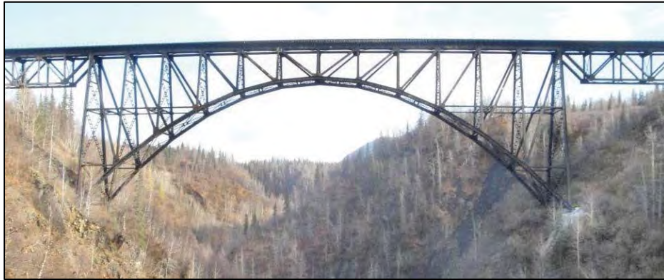
Figure 4-4 Hurricane Gulch Bridge
