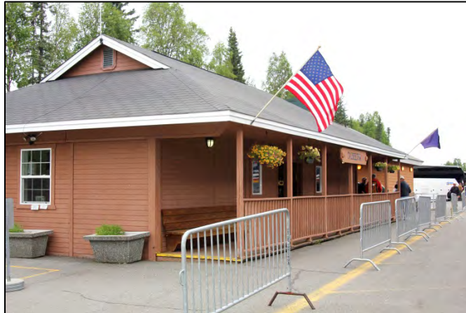
Figure 3-6 Talkeetna Railroad Depot
