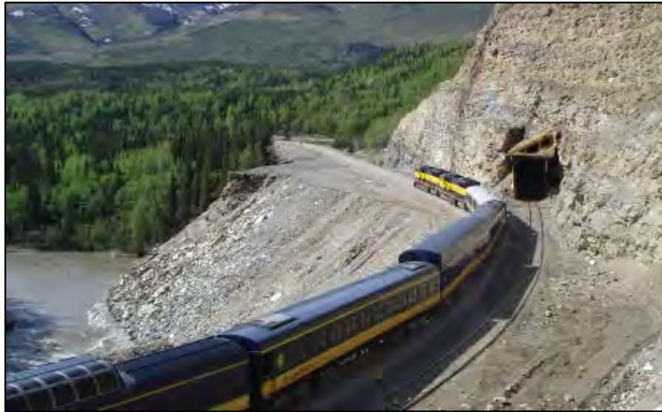
Figure 5-8 Track Realignment near Healy
