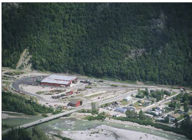
Figure 3-16 WP&YR Maintenance Facility
