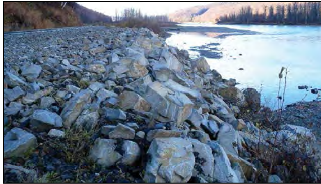
Figure 4-2 Bank Stabilization along the Susitna River
