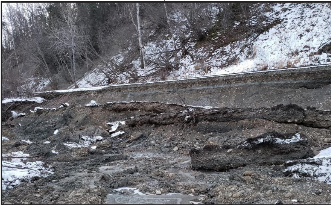
The 2018 earthquake caused extensive shoulder and sub-structure damage to track infrastructure.
