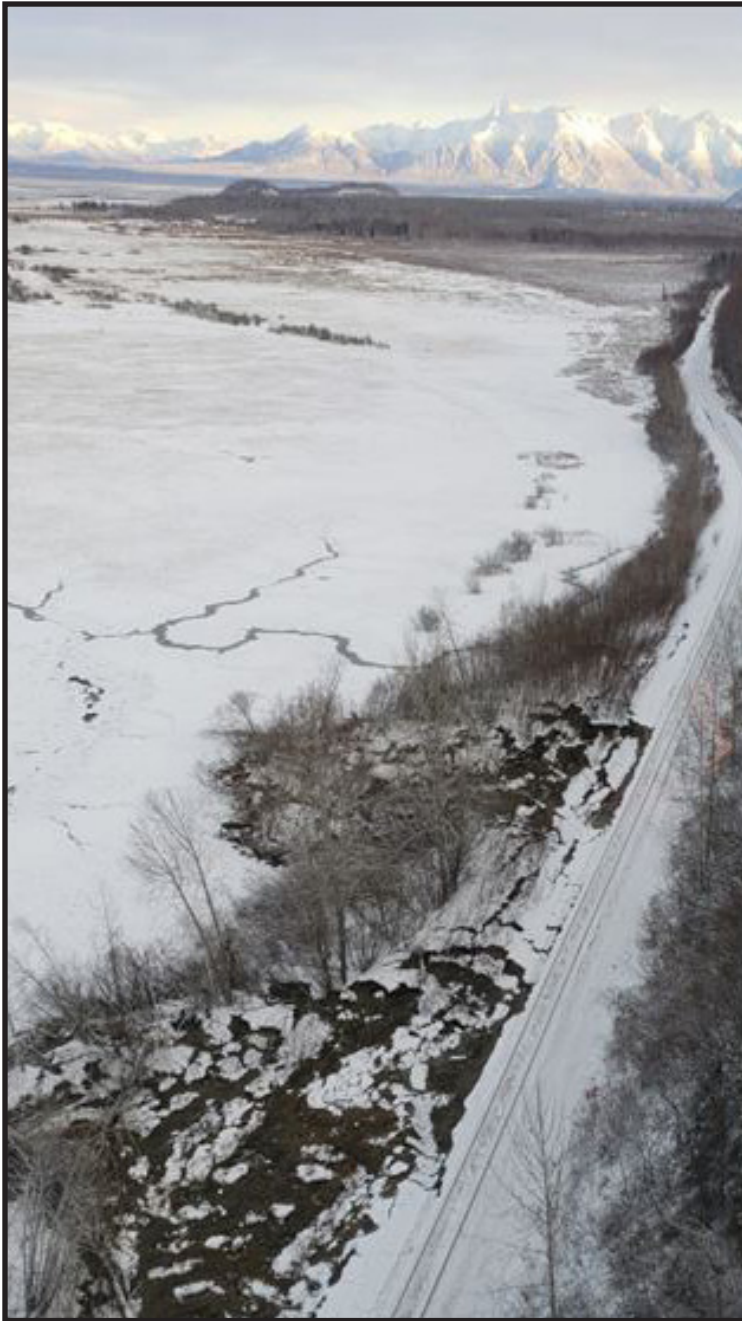
The 2018 earthquake caused shoulder and sub-structure damage along a stretch of track about 25 miles north of Anchorage.
