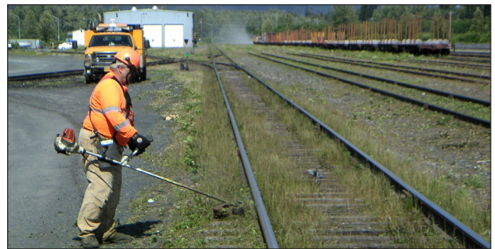
Ineffective mechanical/manual control in Seward yard prior to chemical application.
