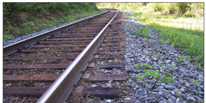
Post herbicide control near Seward. Note clear distinction at control area boundary at end of tie.
