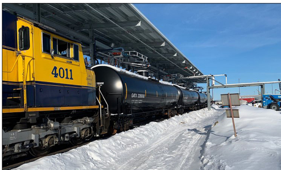
Petro Star's new fuel distribution system came on line in 2020, with terminals in Anchorage (pictured) and Fairbanks.
