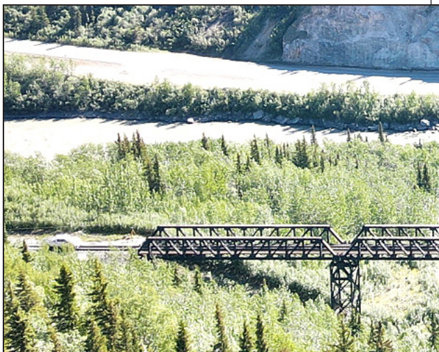
Top-right: The triple-span pony truss bridge at MP 351.4 will be replaced with a triple-span deck plate girder bridge. Inset photo: Crews weld steel components on a replacement bridge at MP F9.4.
