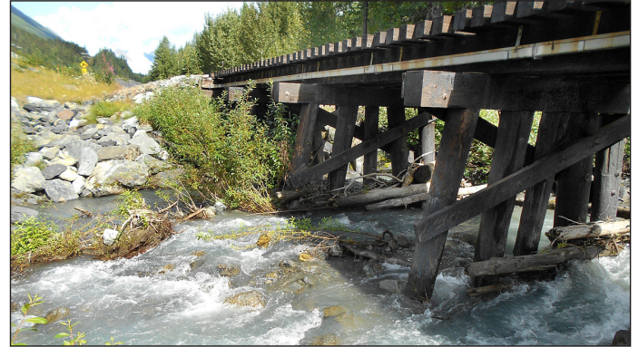
Above: The timber trestle bridge at MP 25.4 over Falls Creek is being replaced with a four-span concrete ballast deck bridge (see drawing at left for reference).
