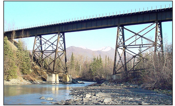
The deck girder bridge at MP 127.5 over Eagle River will be replaced with a deck plate girder bridge.
