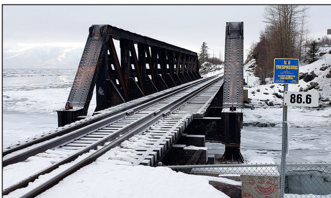
Above: The pony truss and timber trestle bridge at MP 86.6 over Bird Creek will be replaced with a bridge comprised of two steel beam spans and a thru-plate girder span (see drawings at right for reference).
