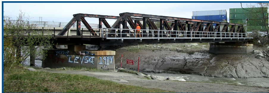
Bridge at Milepost 114.3.
