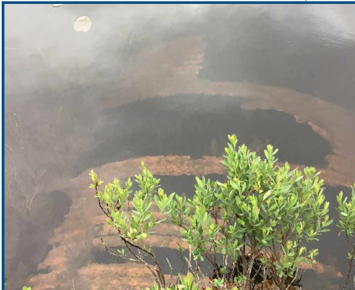
Culvert (underwater) located at MP 66.09 showing extensive wear and corrosion.
