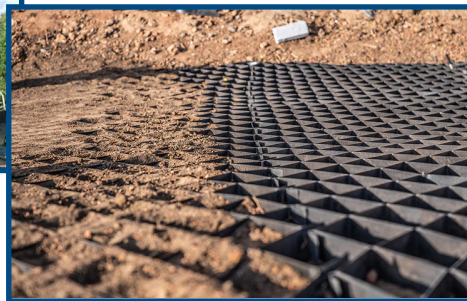
Right: Example of geogrid that will be used for stabilization.
