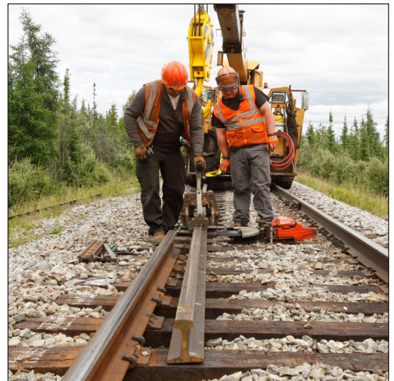
Left: A tie crane operator positions a new tie during tie replacement operations. Right: Rail replacement operations. (Photos by Judy Patrick)
