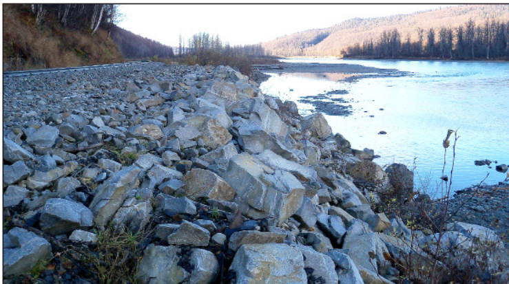
Rip-rap and armor rock are placed along the Susitna River.
