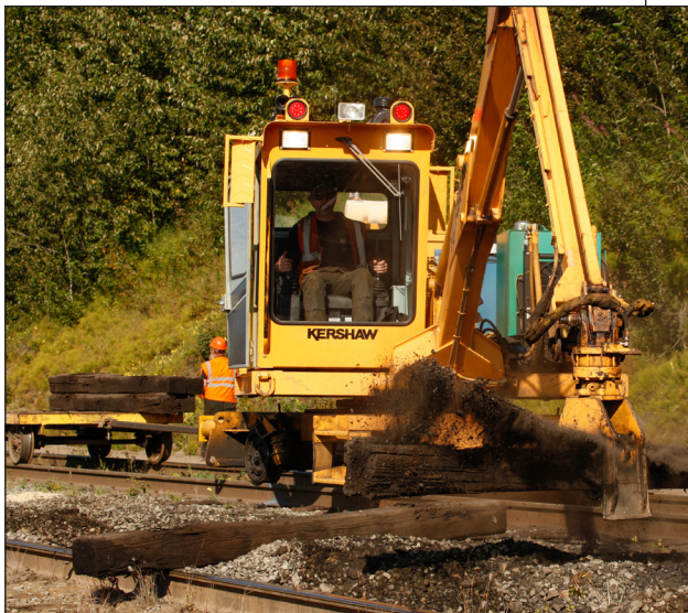
Left: A tie crane operator positions a new tie during tie replacement operations. Right: Rail replacement operations. (Photos by Judy Patrick)
