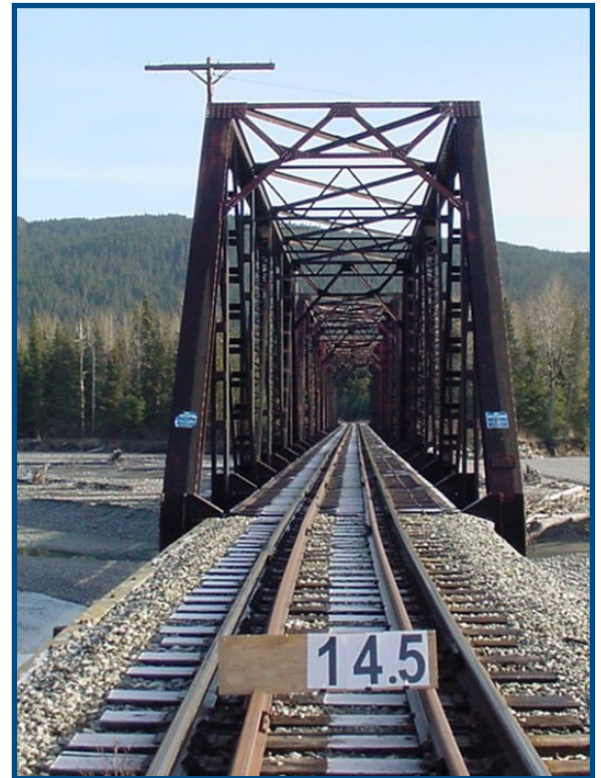
Bridge 14.5 will have the tie deck replaced, replace broken rivets with high strength bolts and install a trainman's walkway for maintenance personnel safety.
