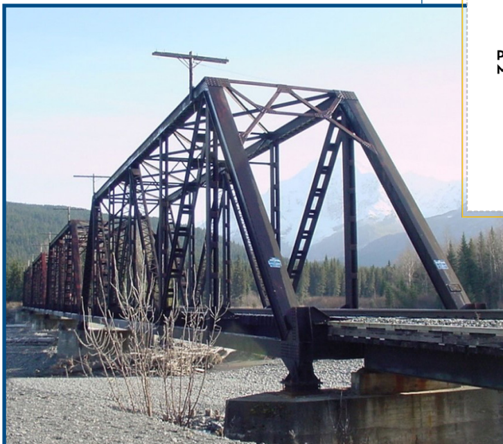
Bridge 14.5 crosses the Snow River. Rehabilitation plans for the bridge includes removal of two existing spans from the southern approach.
