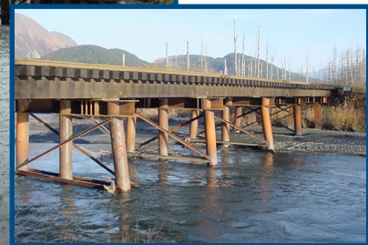
Bridge 3.7 crosses Salmon Creek in Seward, Alaska. The project will include replacing the existing seven (7) 15-foot timber spans with four (4) new SBD bridge spans.
