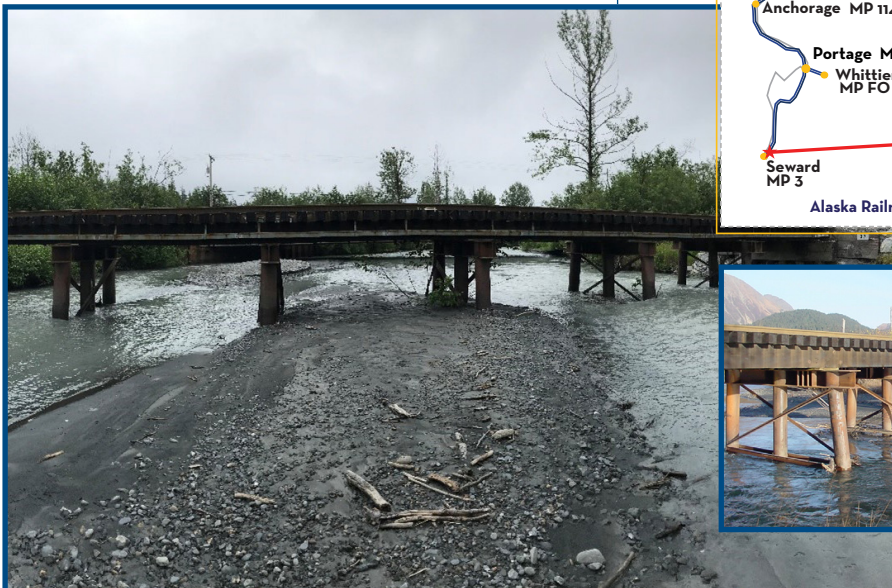
Bridge 3.7 crosses Salmon Creek in Seward, Alaska. The project will include replacing the existing seven (7) 15-foot timber spans with four (4) new SBD bridge spans.
