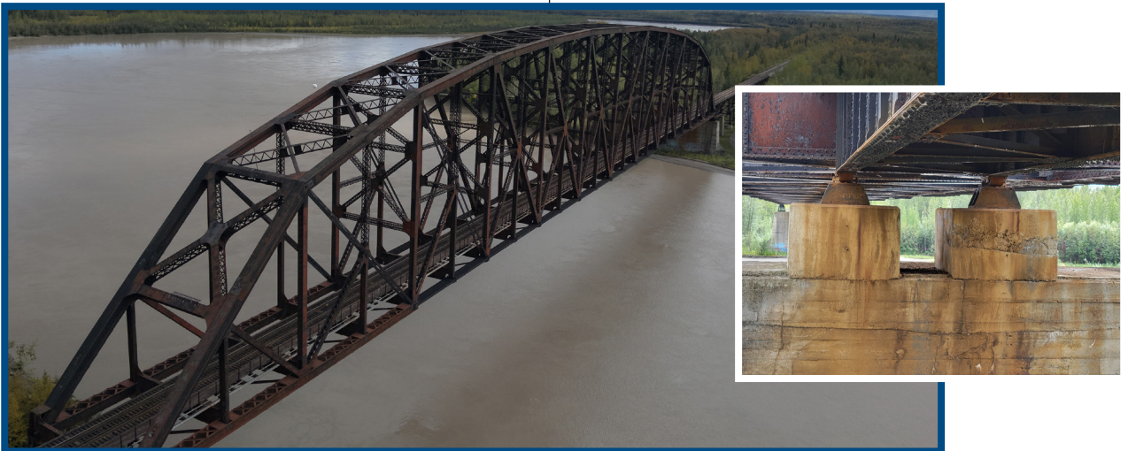
Above: ARRC received an FRA CRISI (Consolidated Rail Infrastructure And Safety Improvements) Program grant to rehabilitate this 1,298-foot, 12-span through truss bridge over the Tanana River in Nenana, Alaska (MP 413.7).
