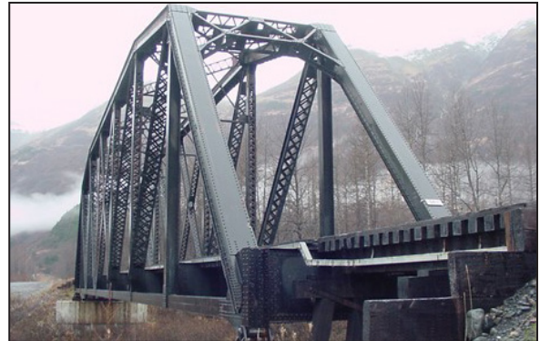
Above: The bridge at MP 54.1 over the Placer River near Spencer Glacier is being rehabilitated, including replacing four (4) 15-foot timber approach spans and abutments with two (2) steel beam spans and abutments.
