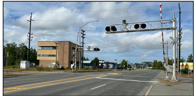
Crossing at Spenard Road in Anchorage.
