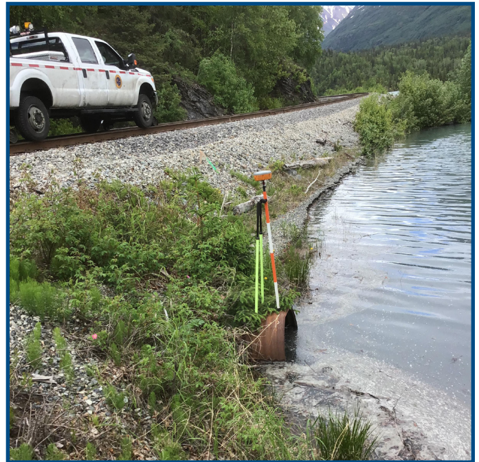
Culvert located at MP 26.2.
