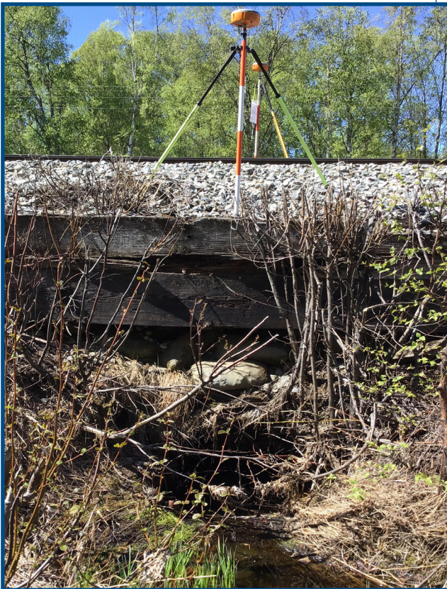
Culvert located at MP 225.97 near Talkeetna Depot.
