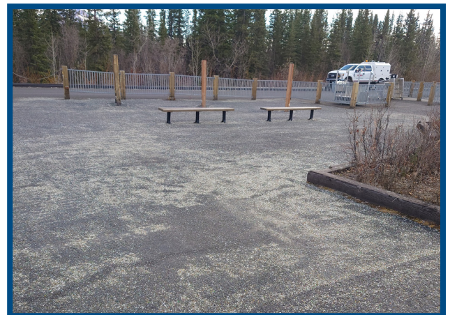
Asphalt visibly sheds glass shards due to asphalt degradation.
