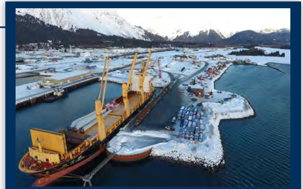
Photo III-1.12: Freight Dock (Source: lukedavisphotography.smugmug.com, 2017)
