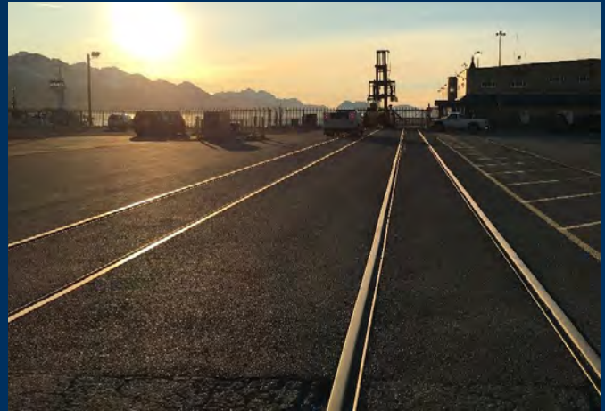
Photo III-1.9: Passenger Dock Tracks (Photo: Hanson, 2015)
