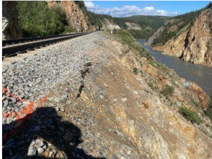
Photo of Approach to Wall Start Looking Up Station
