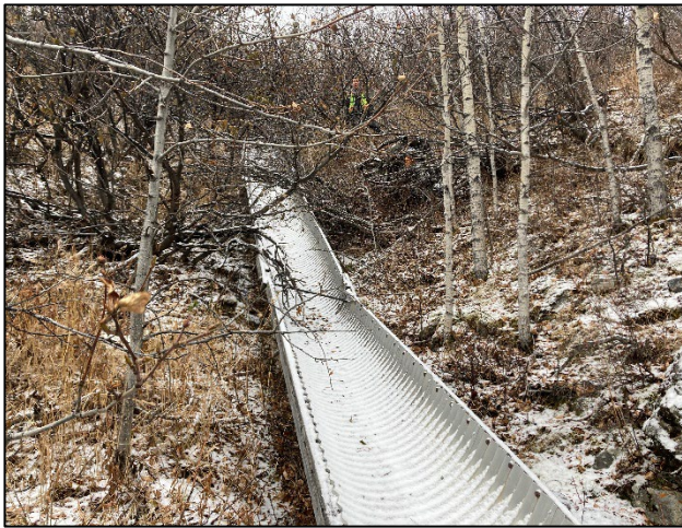
Photo 2.1: Existing flume west of the tracks, looking south
