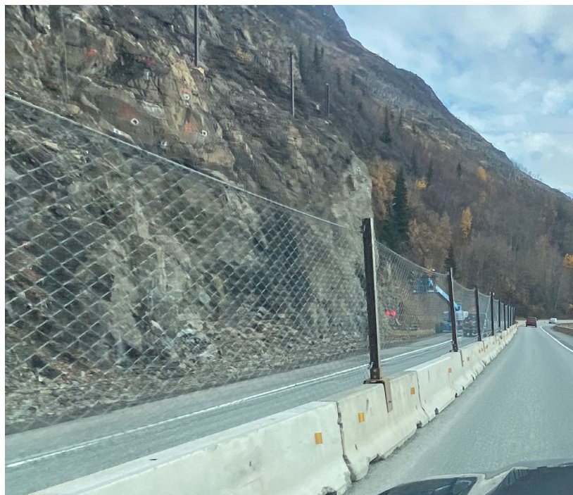
Figure 5.2: Jersey Barrier with Fencing
