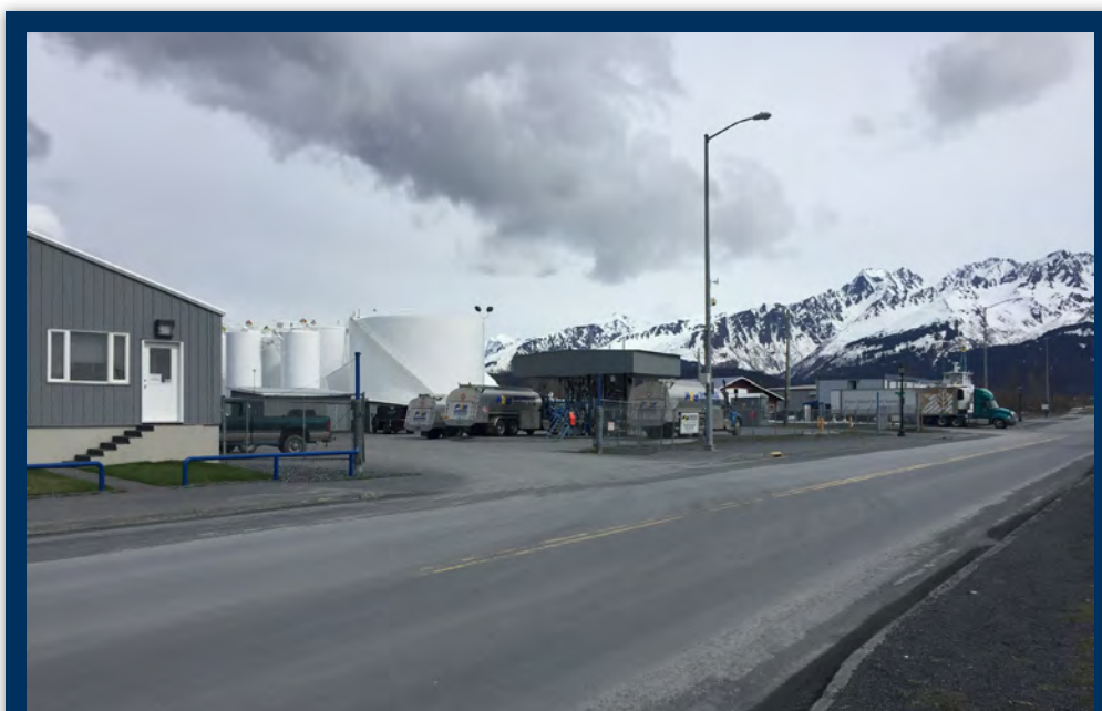
Photo 2-12: Petroleum Facilities (Source: DOWL, 2017)
