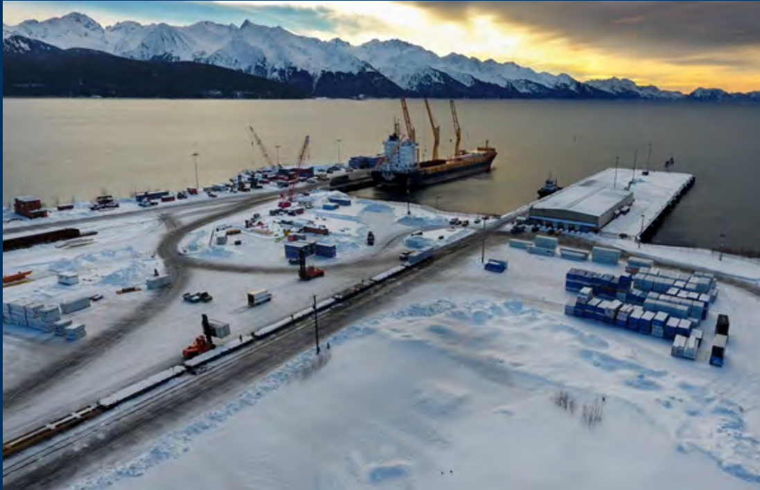
Photo 2-8: Permit and Laydown Areas Inside Freight Dock Fence (Source: lukedavisphotography.smugmug.com, 2017)
