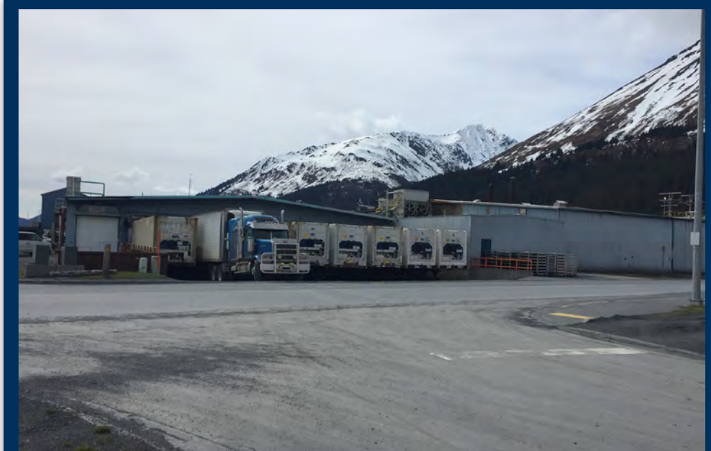
Photo 2-11: Fish Processing Facilities (Source: DOWL, 2017)
