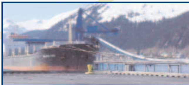
The facility conveyor discharges coal into a ship's hold.
