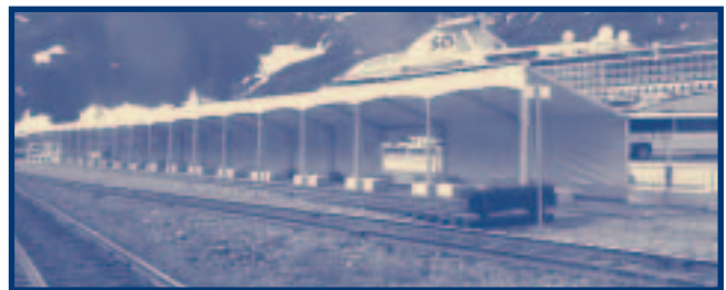
Whittier: A shelter is constructed over a path to the train.
