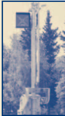
A wayside horn is mounted at Klatt Rd. crossing.
