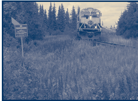
Weeds overrun the mainline track in many locations.
