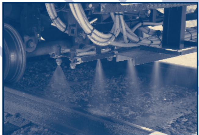
Specialized equipment directs chemical weed control on the track.
