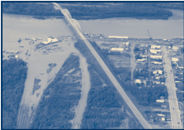
River flooding puts road and rail under water in Nenana.
