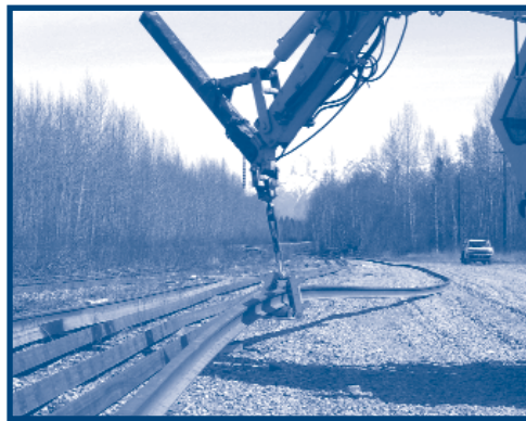
Continuously welded rail reduces maintenance costs and improves passenger ride quality.
